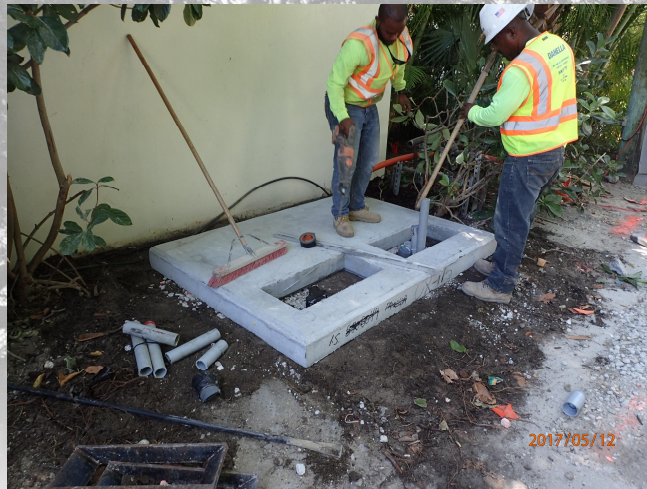
Equipment Pad Installation
