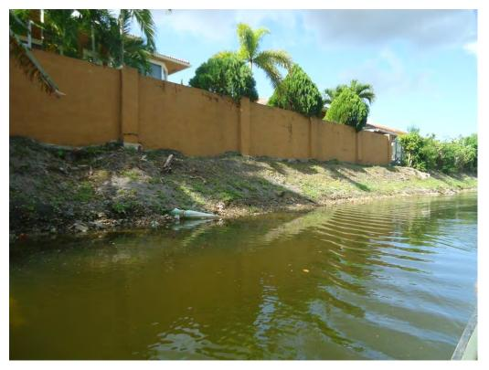
Photo 19. Canal Section 2.3 – View is to Southwest, showing minor slope erosion.
