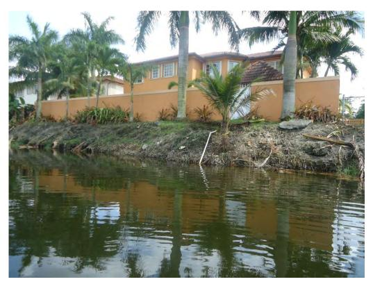
Photo 31. Canal Section 3.9 – View is to South, showing minor slope erosion.
