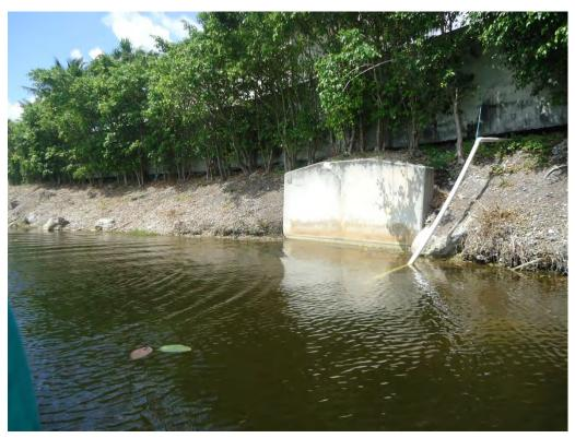
Photo 41. Canal Section 4.3 – View is to west, showing storm water outfall structure.
