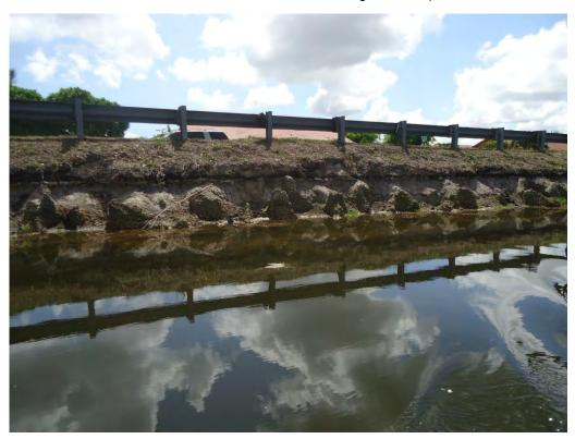
Photo 38. Canal Section 4.2 – View is to East, showing severe slope erosion.
