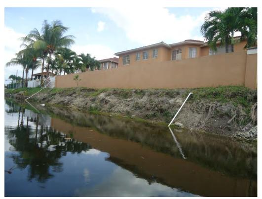
Photo 32. Canal Section 3.10 – View is to South, showing some slope erosion.
