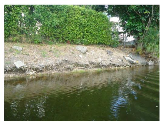
Photo 40. Canal Section 4.3 – View is to East, showing concrete debri on canal slope.
