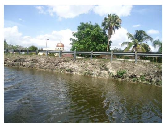
Photo 42. Canal Section 4.3 – View is to East, showing some to severe slope erosion.
