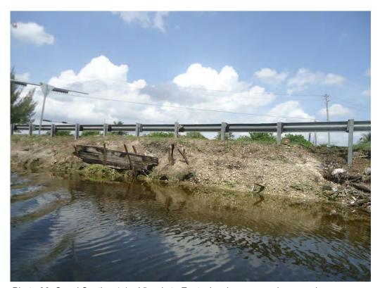
Photo 36. Canal Section 4.1 – View is to East, showing severe slope erosion.
