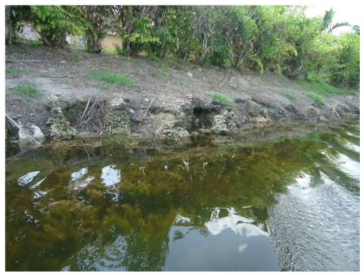
Photo 37. Canal Section 4.2 – View is to west, showing some slope erosion.
