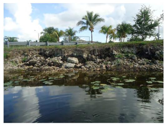
Photo 9. Canal Section 1.7 – View is to North, showing severely eroded slope.
