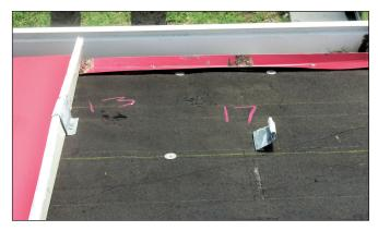
Figure 4. These eave clips were too far from the panel ends. The clip at the left was 13" from the edge of the deck. The other clip was 17" from the edge. It would have been prudent to install double clips along the eave.
