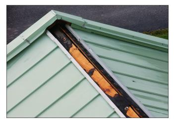
Figure 9. The ridge flashing fasteners were placed too far apart. A significant amount of water leakage can occur when ridge flashings are blown away.
