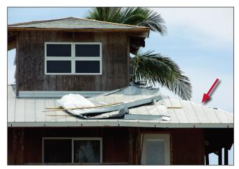
Figure 5. The panels blew off the upper roof and landed on the lower roof of this house. The upper asphalt shingle roof shown had been re-covered with 5V-Crimp panels that were screwed to nailers. The failure was caused by inadequate attachment of the nailers (which had widely-spaced nails) to the sheathing. Note that the hip flashing on the lower roof blew off.
