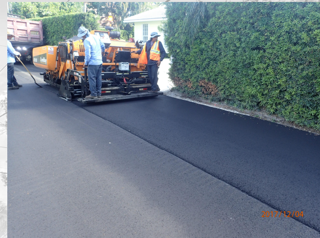
Pavement Restoration/Pole Removal
