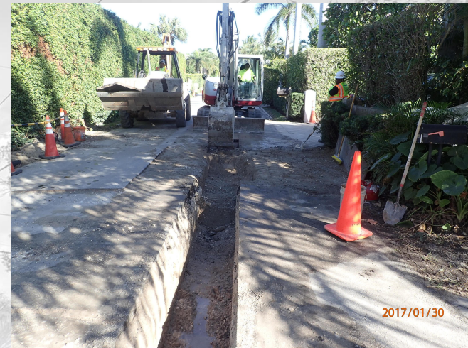
Open Cut Trench
