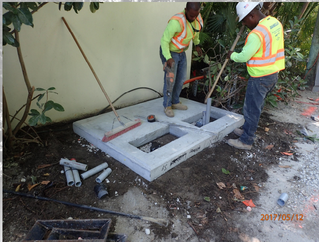
Equipment Pad Installation
