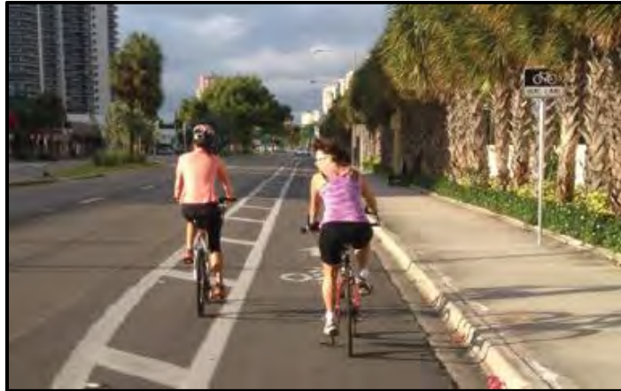
Figure 10: Buffered Bike Lane - Striping
