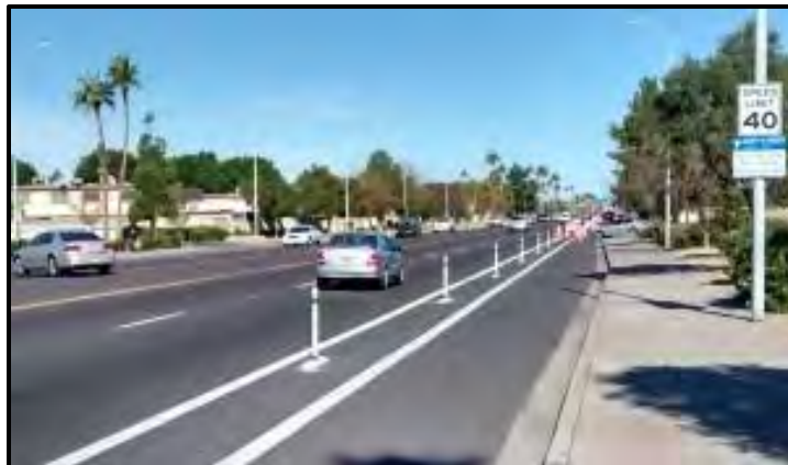
Figure 11: Barrier Separated Bike Lane – Delineators/Flexposts
